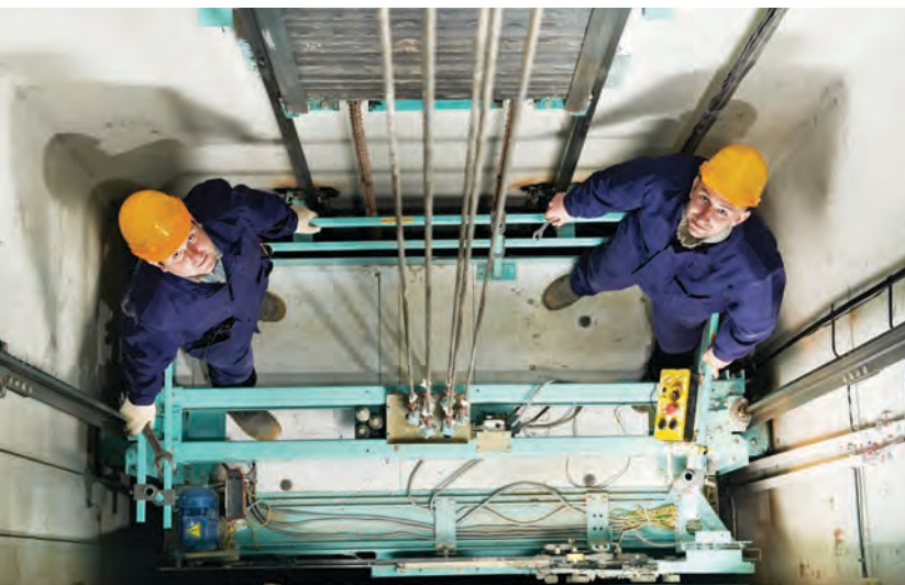
Figure 1.17 Elevator repair is a possession processing service
